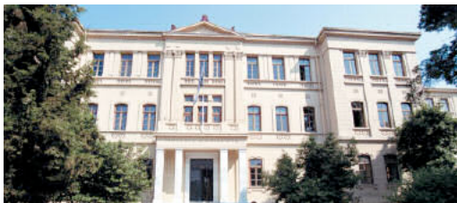
Center for Research and Technology, Greece, (under deployment)
